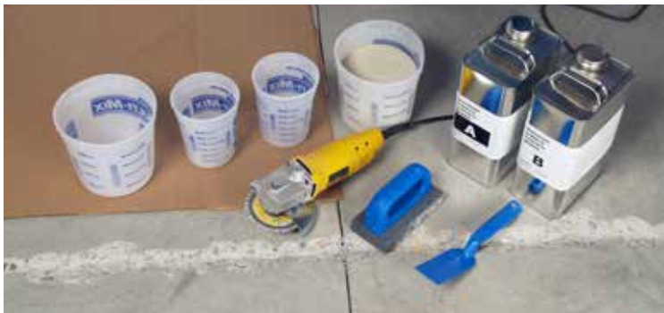
Use bulk to repair spalls and cracks 3/4" or wider.
