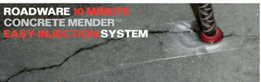
Drill a 3/8" diameter hole about one inch deep into the crack at several points along the crack. Clean the crack and holes with a vacuum.
